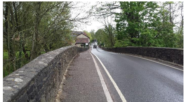
Plate 10: Bridge over the Axe looking southbound
