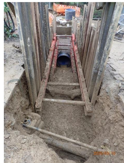
Open Trench with new pipe being installed in the highway at Ivybridge
