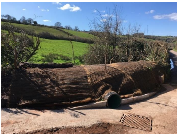
Photographs showing new buddle holes installed on a key surface water flow path into the village. Water taken off the highway into the adjacent field, where the flow will be slowed through a series of NFM interventions.
