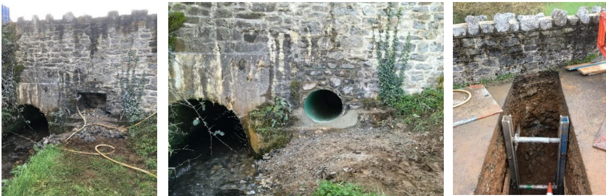
New flood relief culvert being installed in Ugborough
