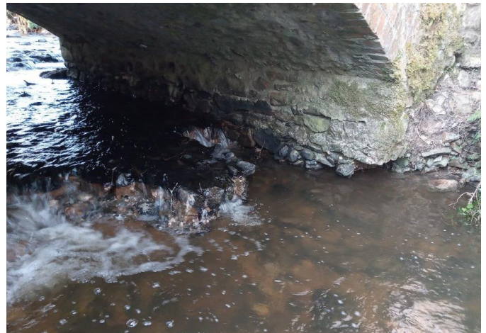
Undermined bridge in need of repair
