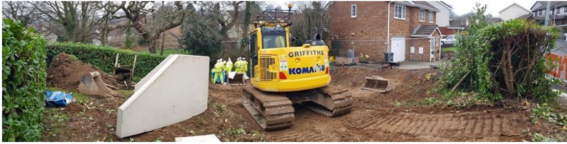
Installation of new outfall in Ivybridge
